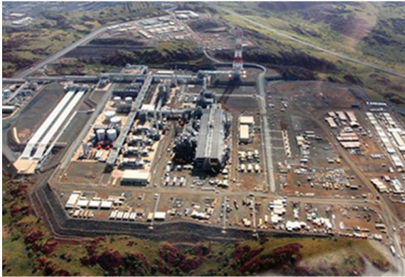
Pluto Gas Plant WA
